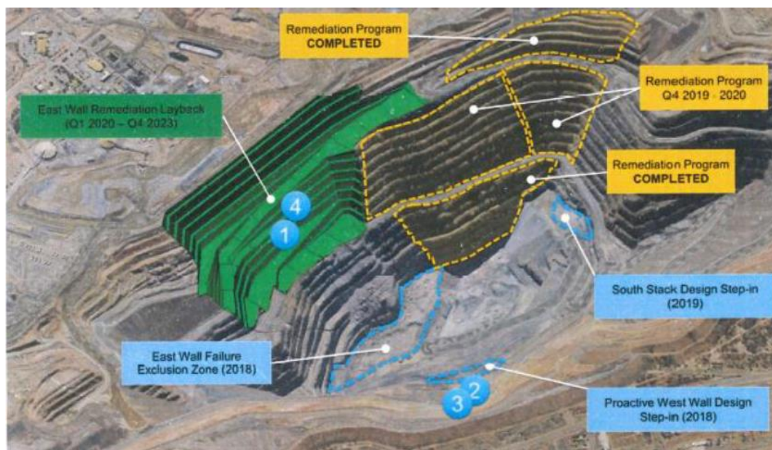
Fig 3 The east wall pit failure showing remediation areas and current exclusion zone
